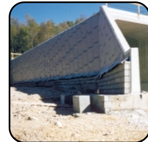
France Cut & cover tunnel
