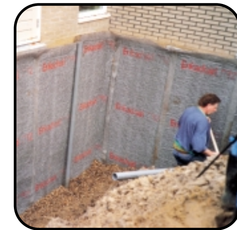
Velp, The Netherlands Basement wall
