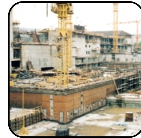
Stuttgart, Germany Lost shuttering
