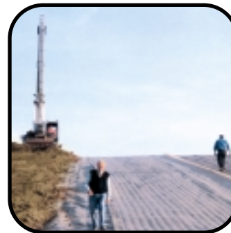
Landgraaf, The Netherlands Water drainage landfill
