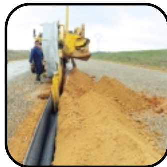
A29, France Road edge drain
