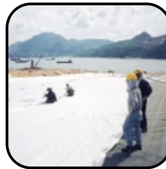
TKO, Hong Kong Water drainage landfill
